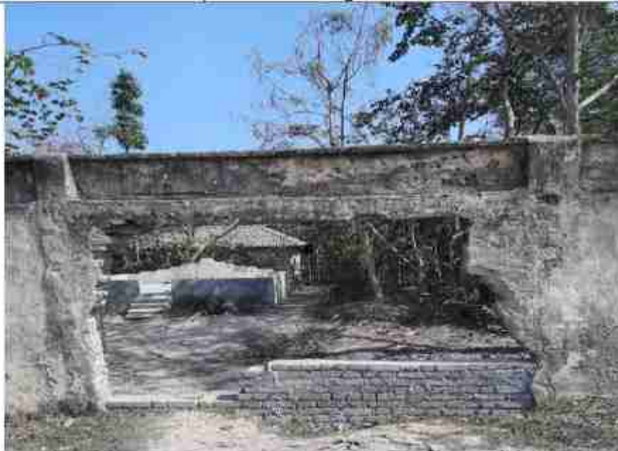
Temple construction under progress in Jethia Village
