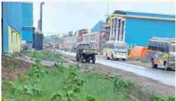
Water sprinkling on road
