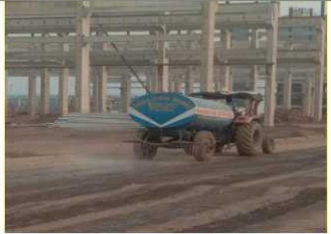
Water sprinkling on road
